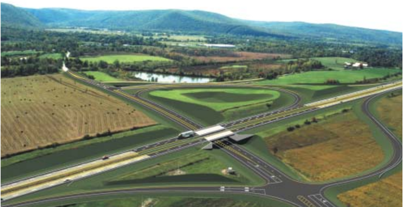
I-86 Interchange #50 is scheduled for completion October, 2003
