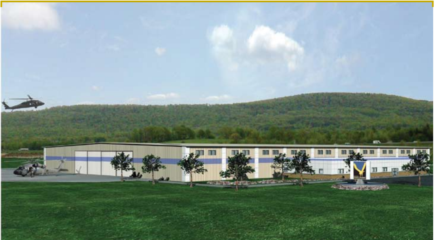
Construction will begin this summer on the new 97,000 square foot Military Derivatives Completion Center at the Elmira Corning Regional Airport in Big Flats, NY.
